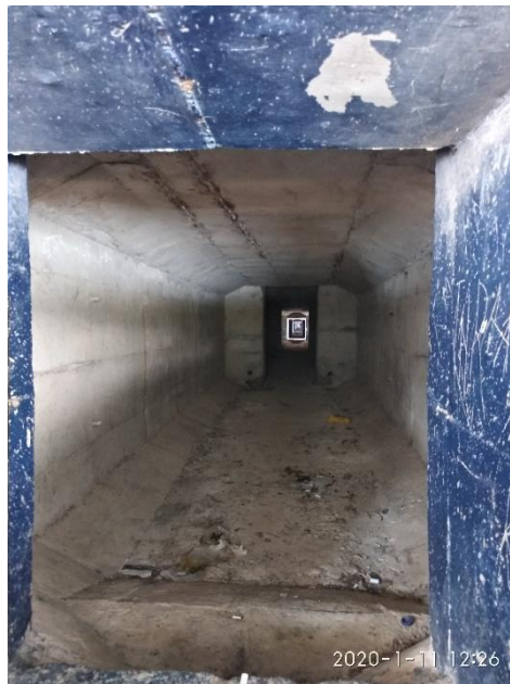
Figure 2. Inside view of PSC Girder of Br.1274 UP between Ullal and Netravathi station
