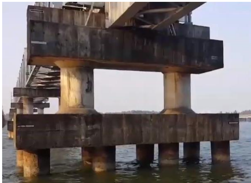
Figure 8. Typical RCC pier of the bridge
