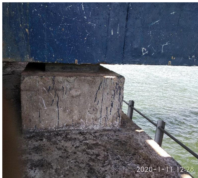
Figure 6. Elastomeric bearing of PSC box girder
