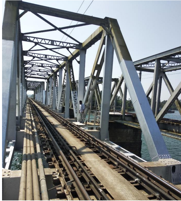
Figure 3. Inside view of the typical Steel truss girder of Br.1274 UP between Ullal and Netravathi Station
