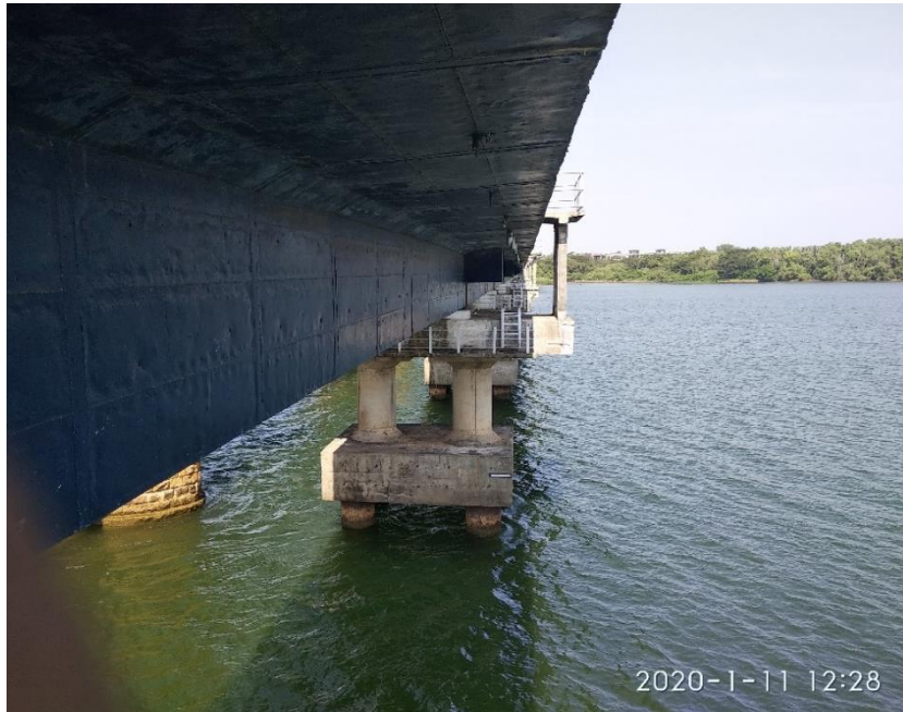
Figure 1. Side view of PSC Girder of Br.1274 UP between Ullal and Netravathi Station
