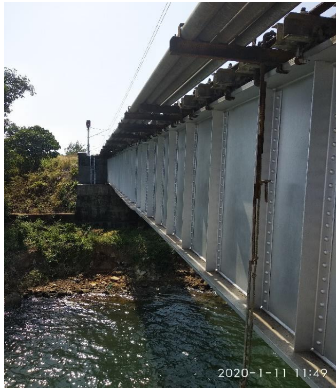
Figure 7. Side view of steel plate girder of Br.1274 UP between Ullal and Netravathi Station
