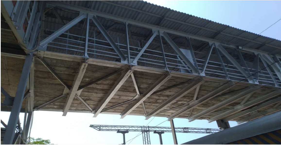
Figure 4. Cross beams and bottom bracing
