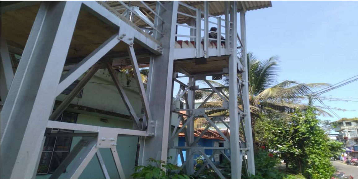
Figure 5. Columns and bracings
