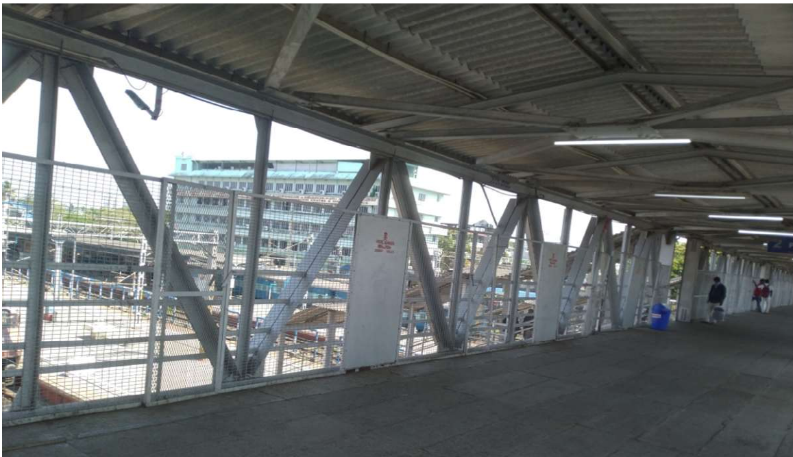
Figure 3. Truss members connected through gusset plates
