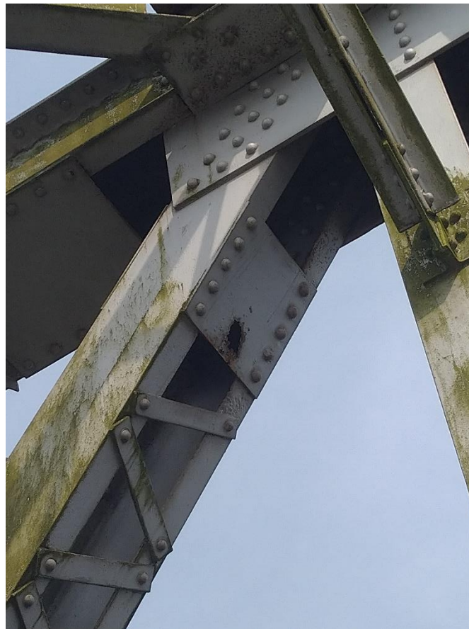
Figure 7. Connection between truss elements
