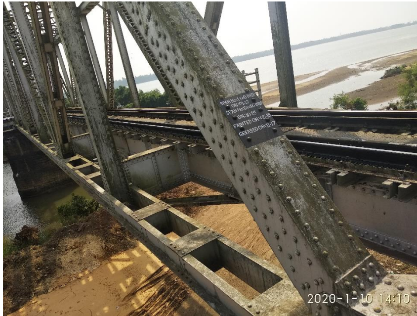
Figure 4. Bottom chord and end diagonal members
