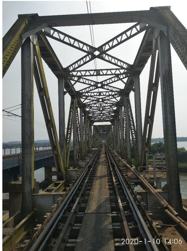
Figure 2. Inside view of the bridge
