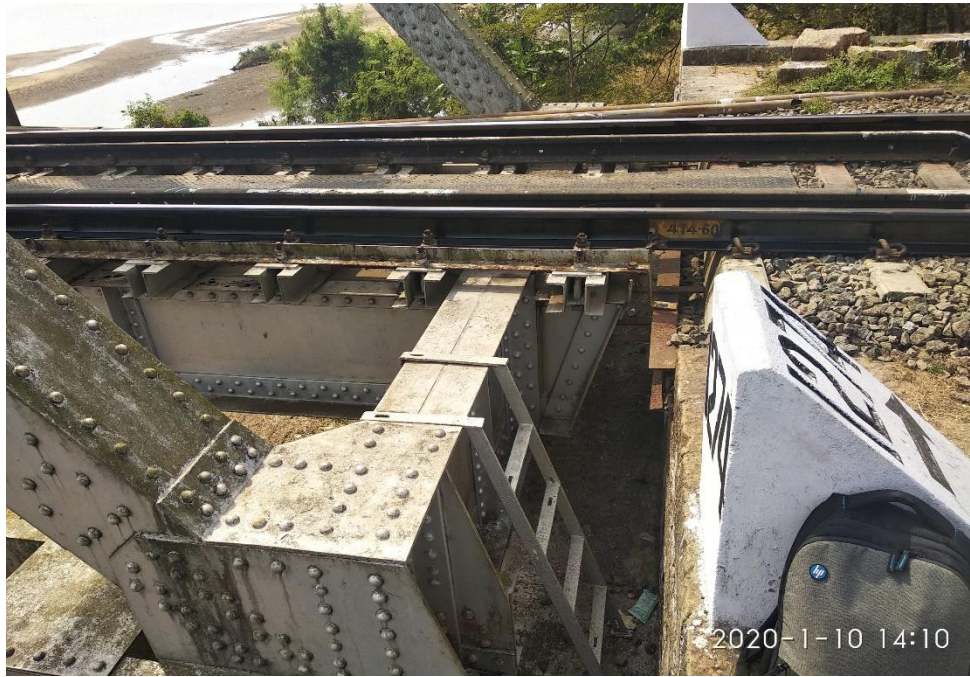
Figure 6. End cross beam
