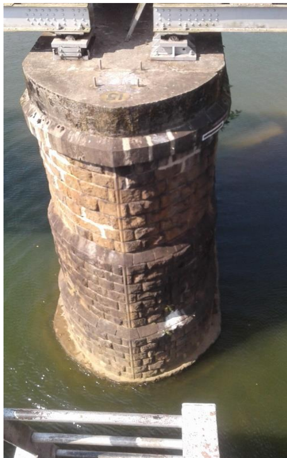
Figure 5. Pier and Bed block
