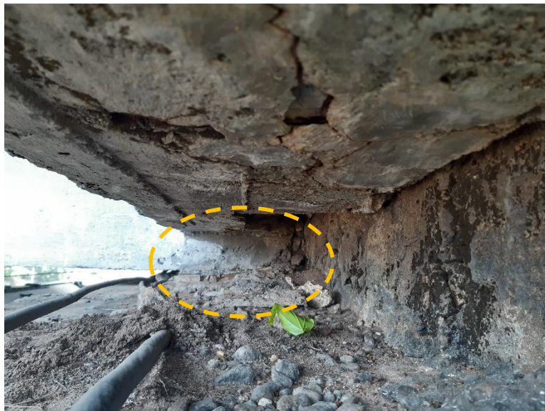
Figure 4. Bearing under girder
