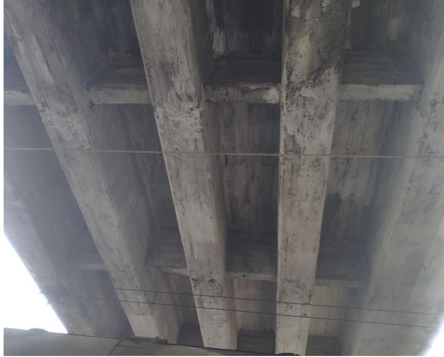
Figure 3. Bottom main beams and Cross beams
