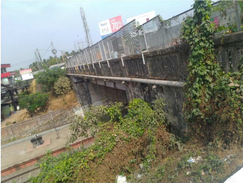
Figure 1. View of Br.872A RCC Bridge
