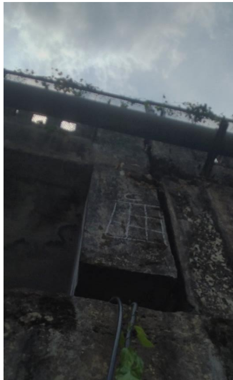
Figure 10. Testing points at Cross girder at western side
