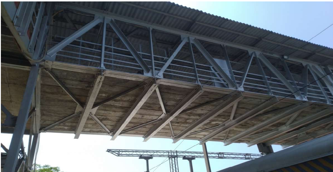
Figure 6. Floor beams and bottom laterals of fourth span
