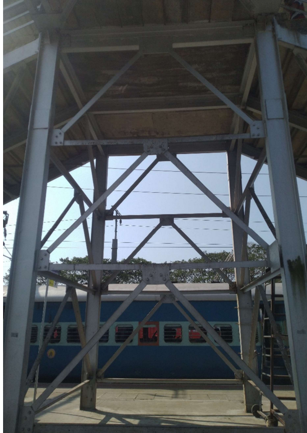
Figure 7. Columns and bracings
