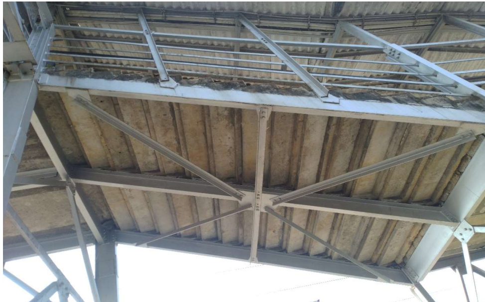
Figure 2. Stair side beams and tie beams
