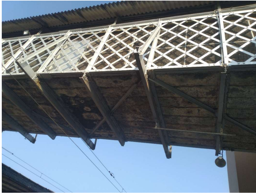
Figure 5. Typical floor beams and bottom laterals of first three spans
