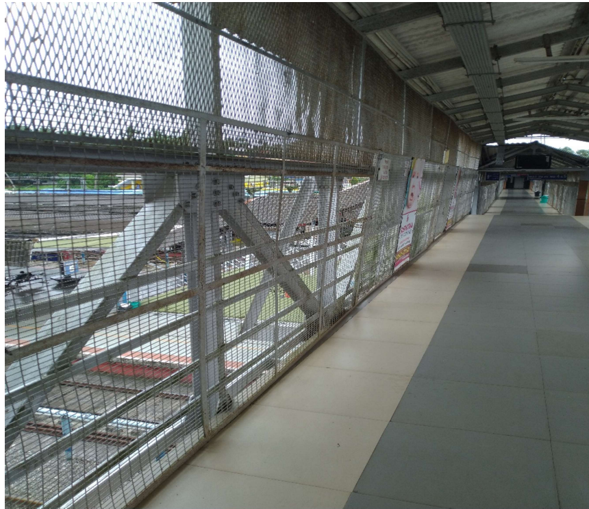
Figure 3. Truss members connected through gusset plates
