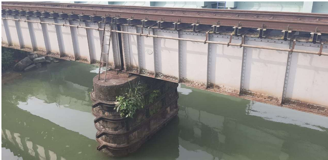
Figure 3. Pier strengthened using rail steel confinement
