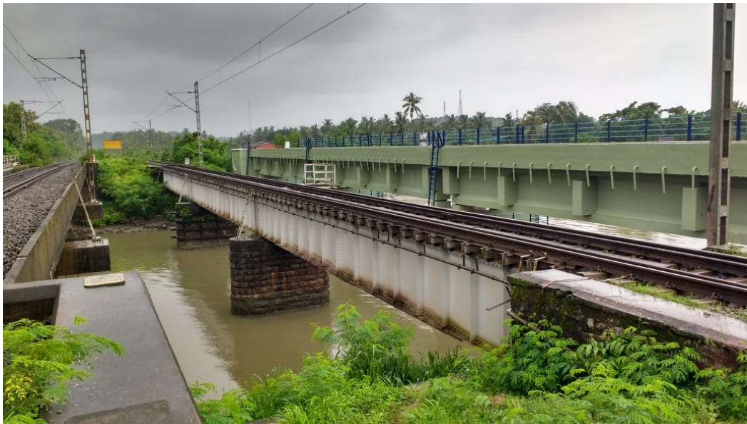
Figure 1. View of Br.1087 Plate girder bridge
