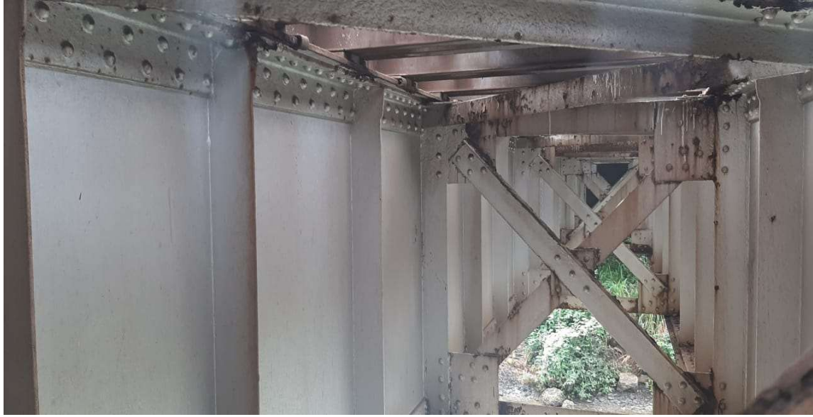
Figure 2. View of the bridge from inside
