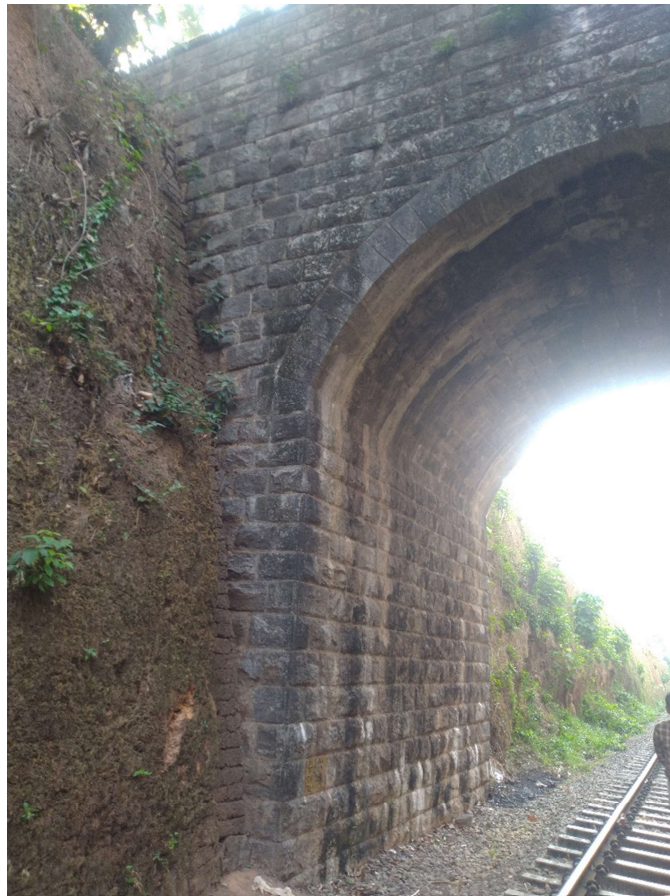
Figure 3. Abutment of the bridge
