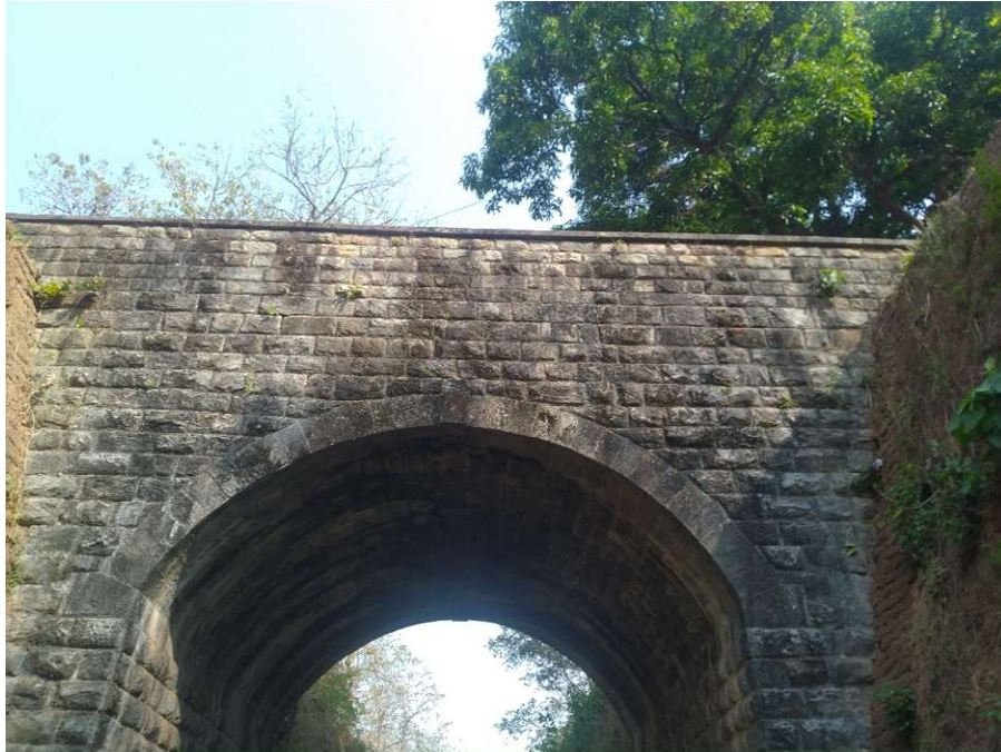
Figure 2. bottom view of the bridge
