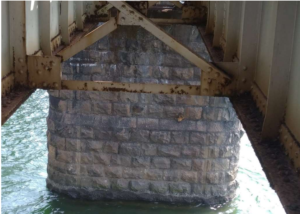
Figure 3. Stone masonry pier
