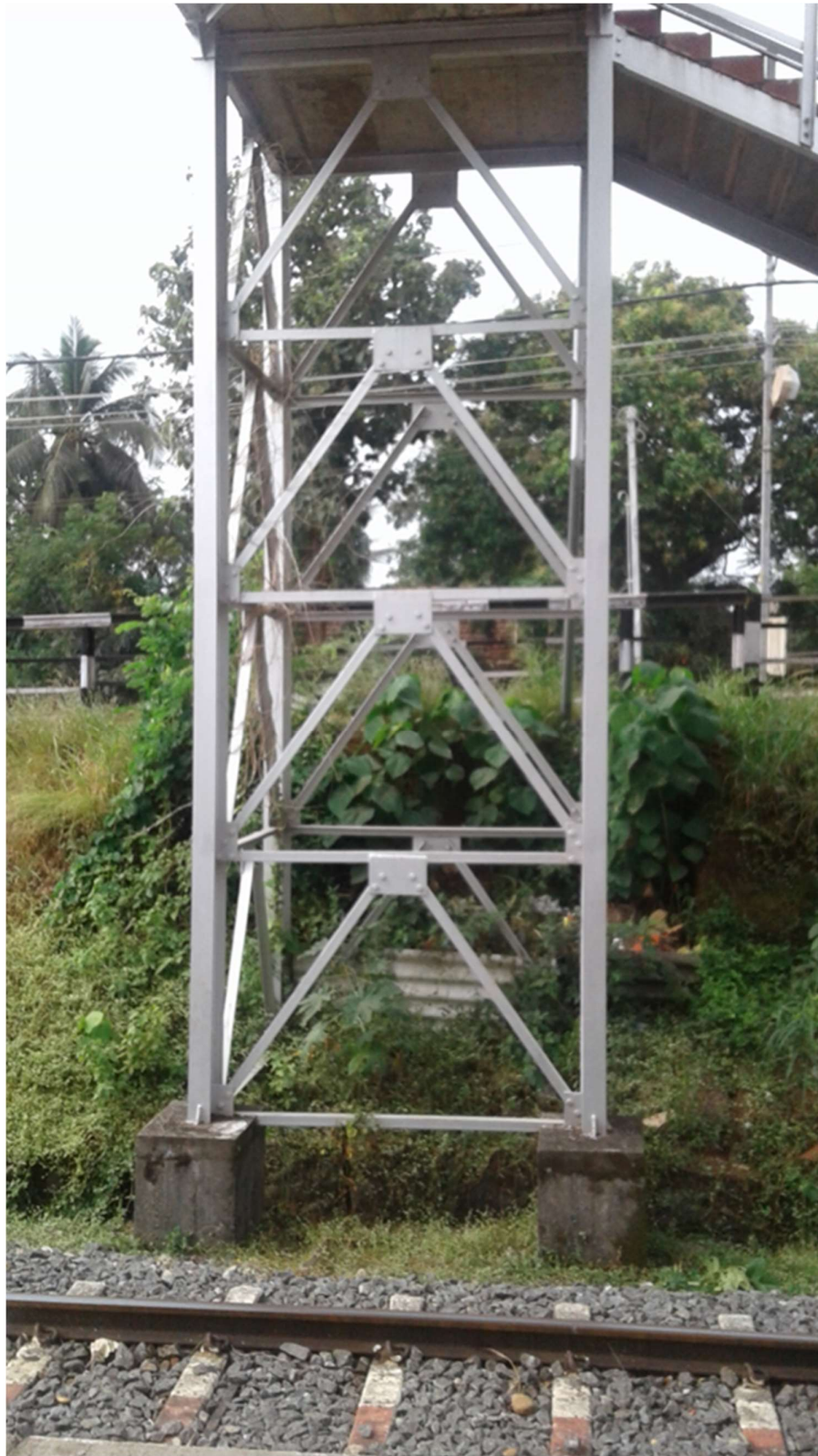
Figure 5. Supporting columns and pedestals
