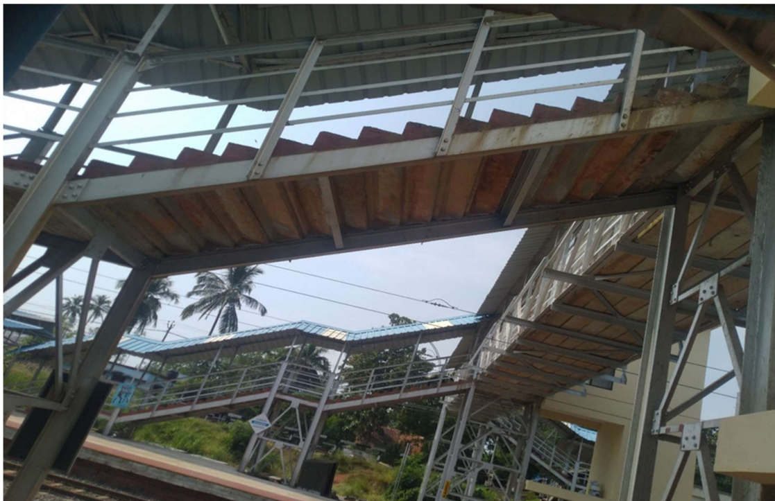
Figure 4. Stair beam and cross beam
