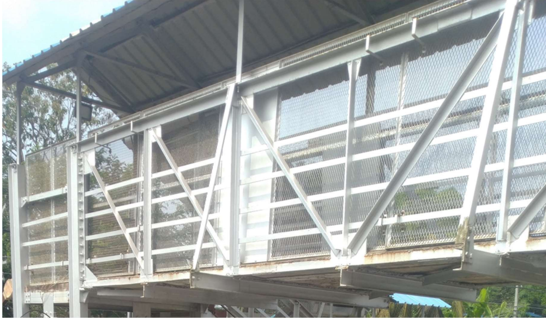
Figure 3. Truss members connected through gusset plates
