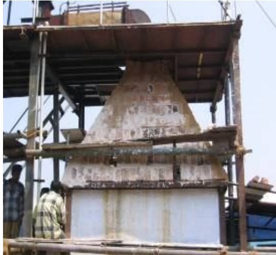
After repair out side view
