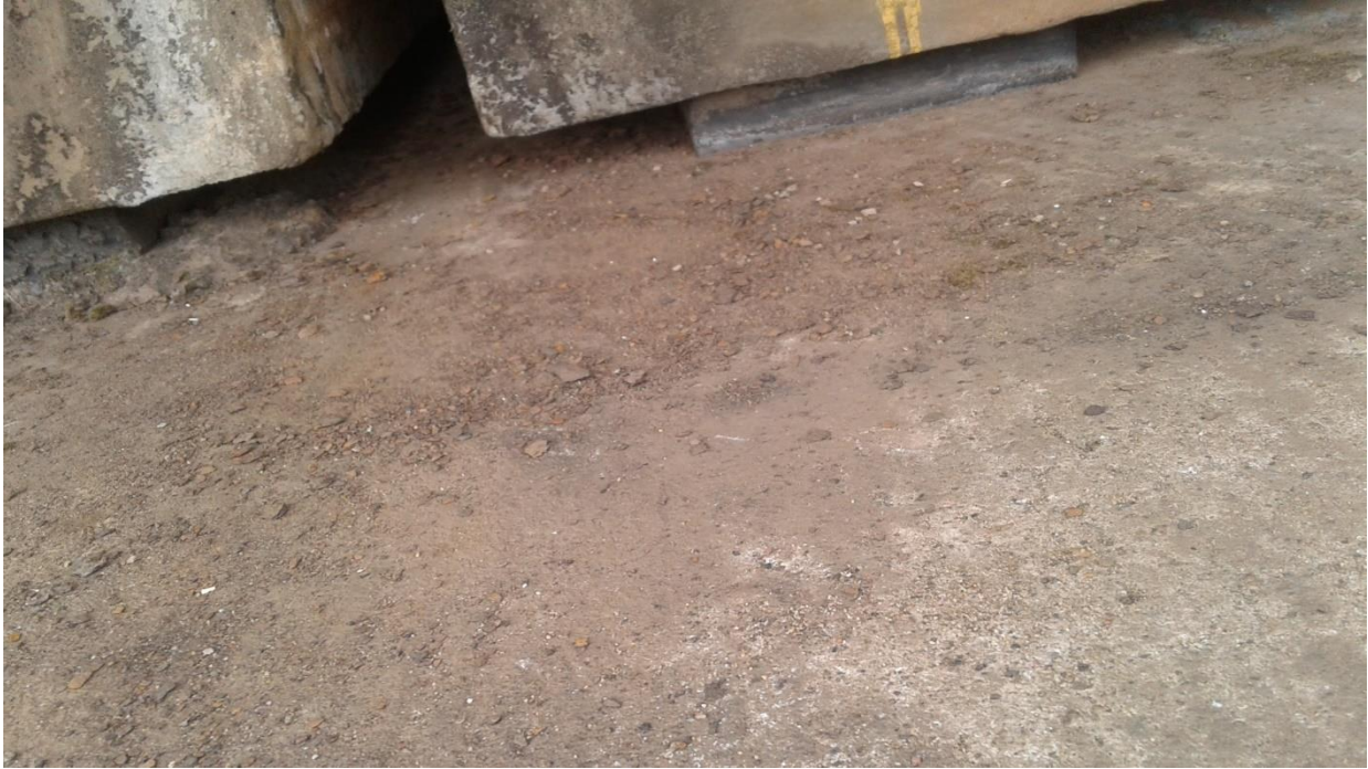
Figure 8 Close view of another bearing
