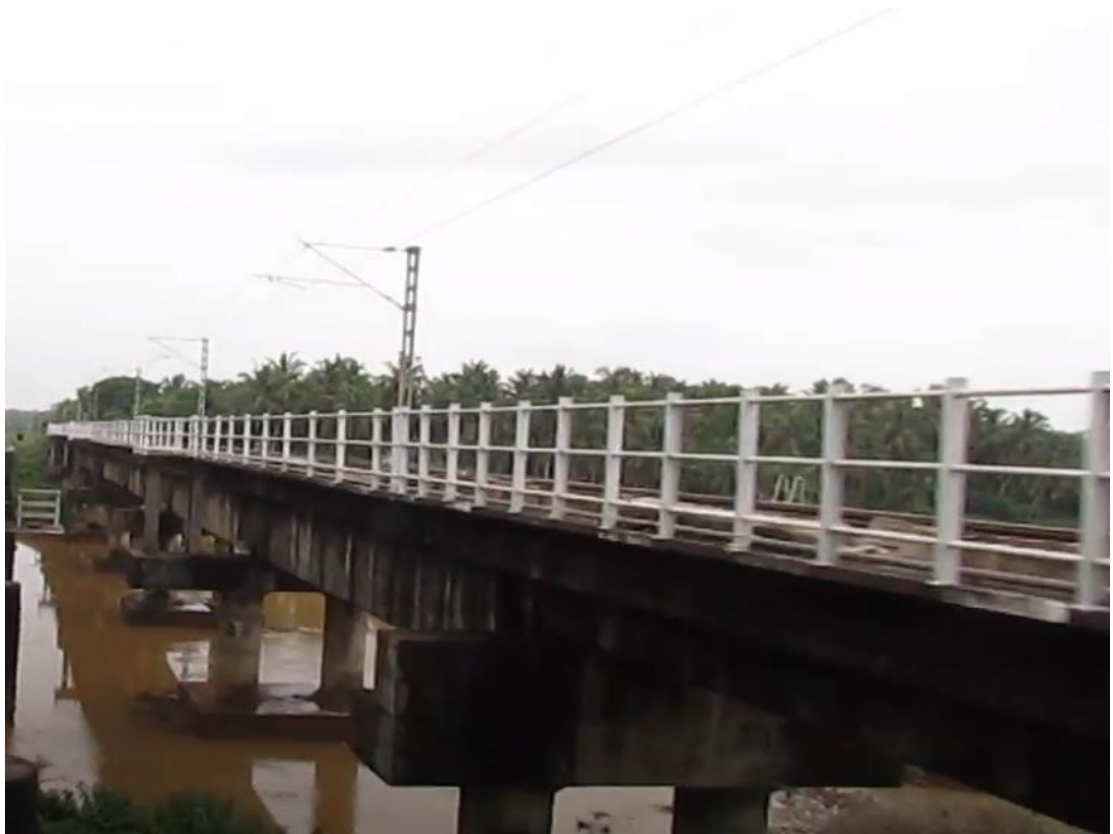
Figure 1. View of Br.1233 DN between Kumbla and Uppala stations
