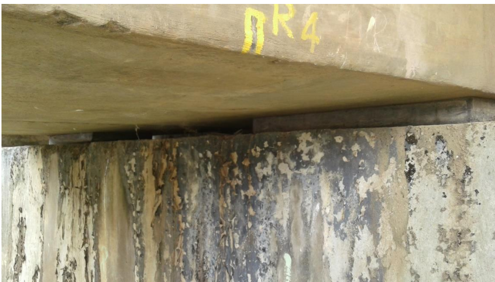
Figure 5 Bearing
