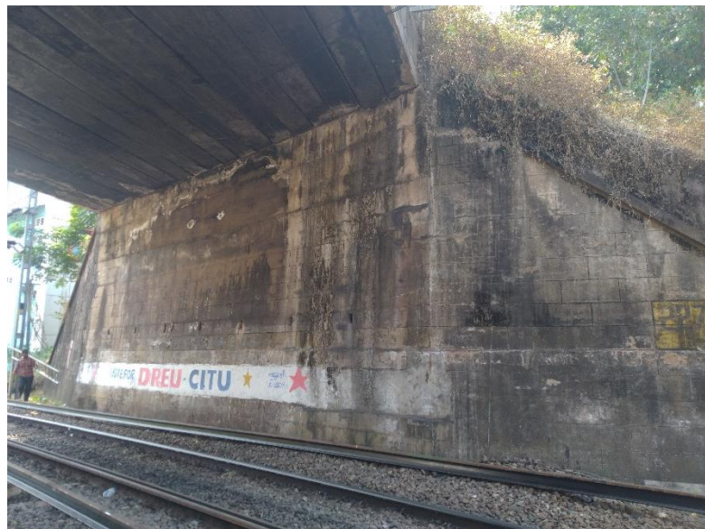
Figure 3. RCC Abutment
