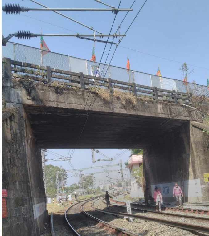
Figure 1. View of Br.2272E Girder type RCC Bridge
