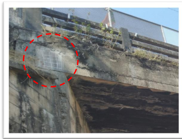
Figure 5. Typical testing point at girder
