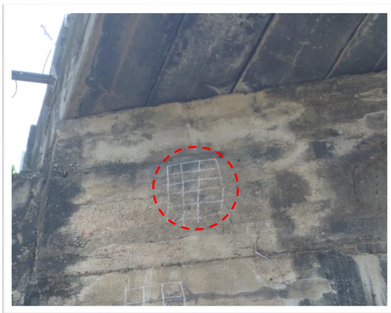
Figure 6. Testing point at top of abutment (Lifted portion)
