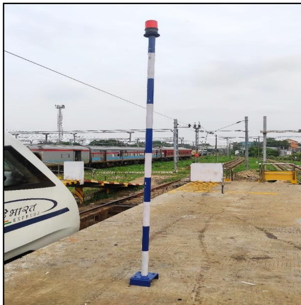
Signal pole installed on east side of pit line No. 3
